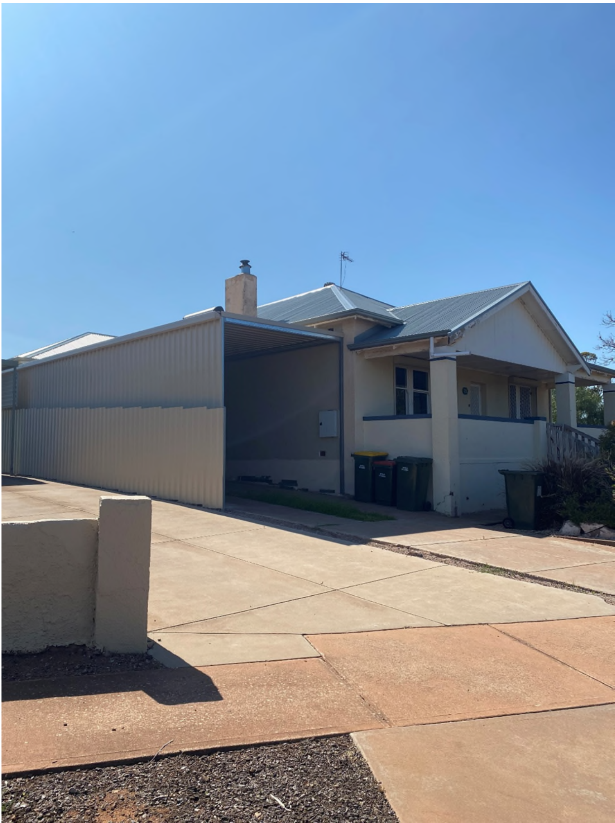
Image 3 – Angled view of structure and associated dwelling
