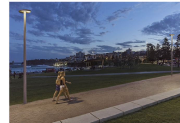
Pedestrian and area lighting.
