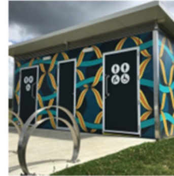
New toilet facilities + amenities.
