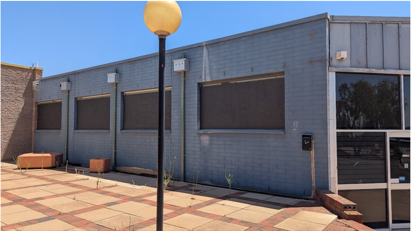
Photo 2: Eastern elevation showing boarded windows – This act does not require assessment
