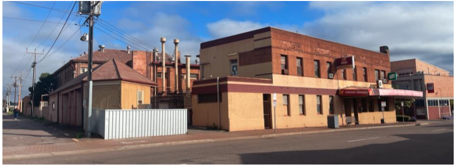
Figure 3: Spencer Hotel, Darling Terrace and Balnaves (rear) Lane frontages . DASH Architects, 2022
