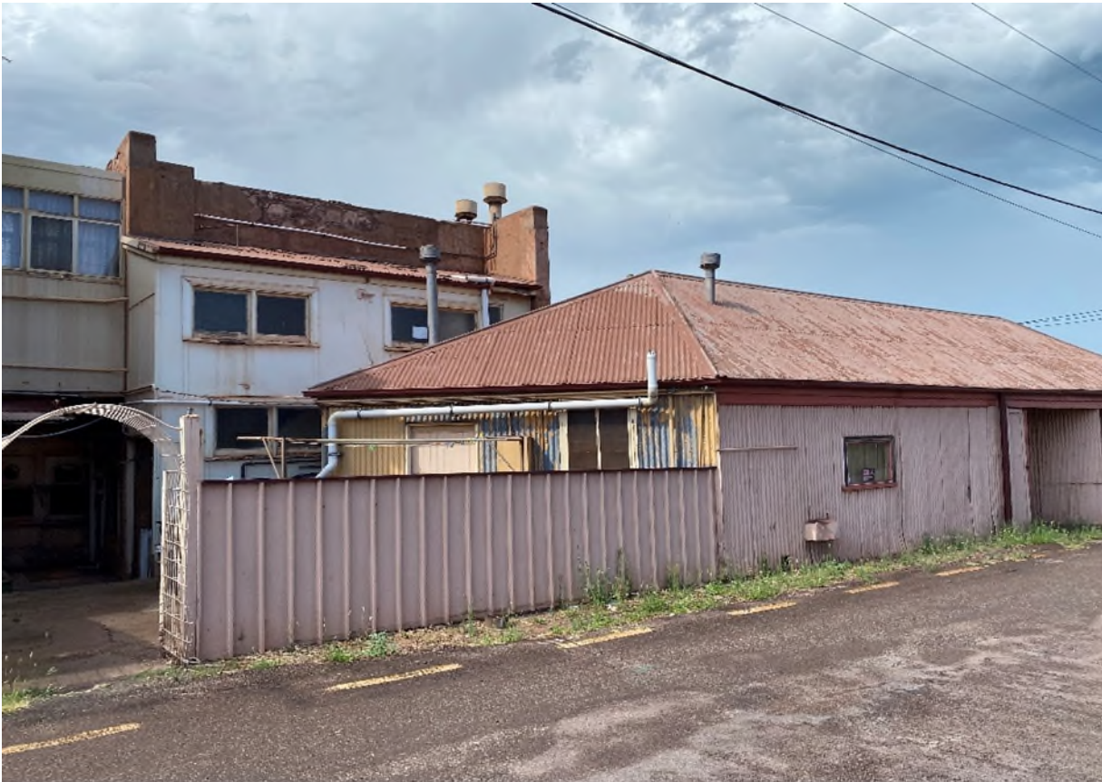
Image 4 – Rear garage for demolition
