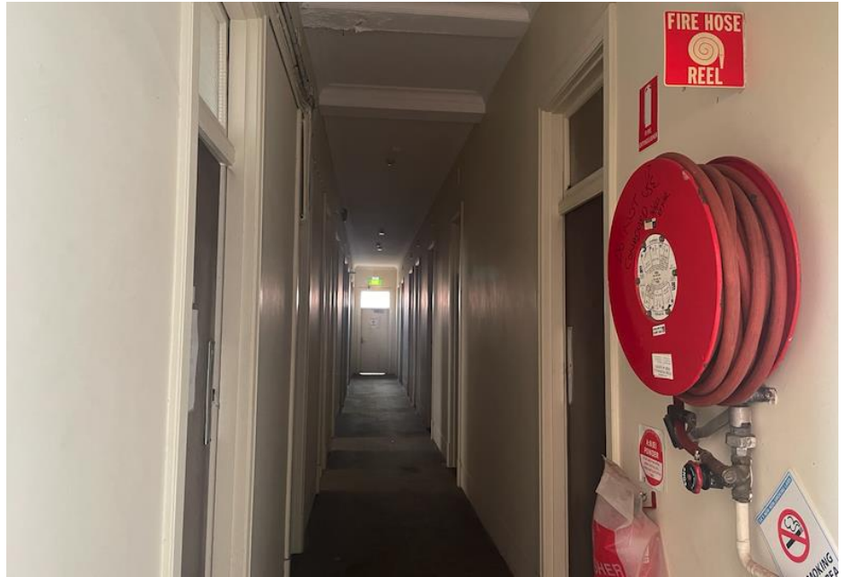
Figure 22: Central corridor of accommodation block. DASH Architects 2022
