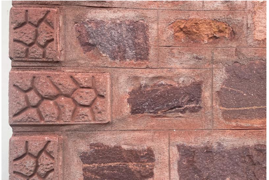
Figure 20: façade detail, showing somewhat crude pressing into stone quoins to replicate a vermiculated carving. DASH Architects, 2022
