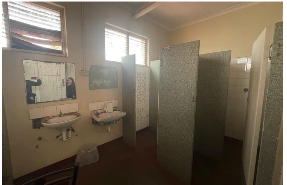
Figure 23: Shared bathroom within accommodation block. DASH Architects 2022
