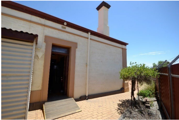
Figure 4: General view of rear entry to Former Customs House with non-complying step ramp
