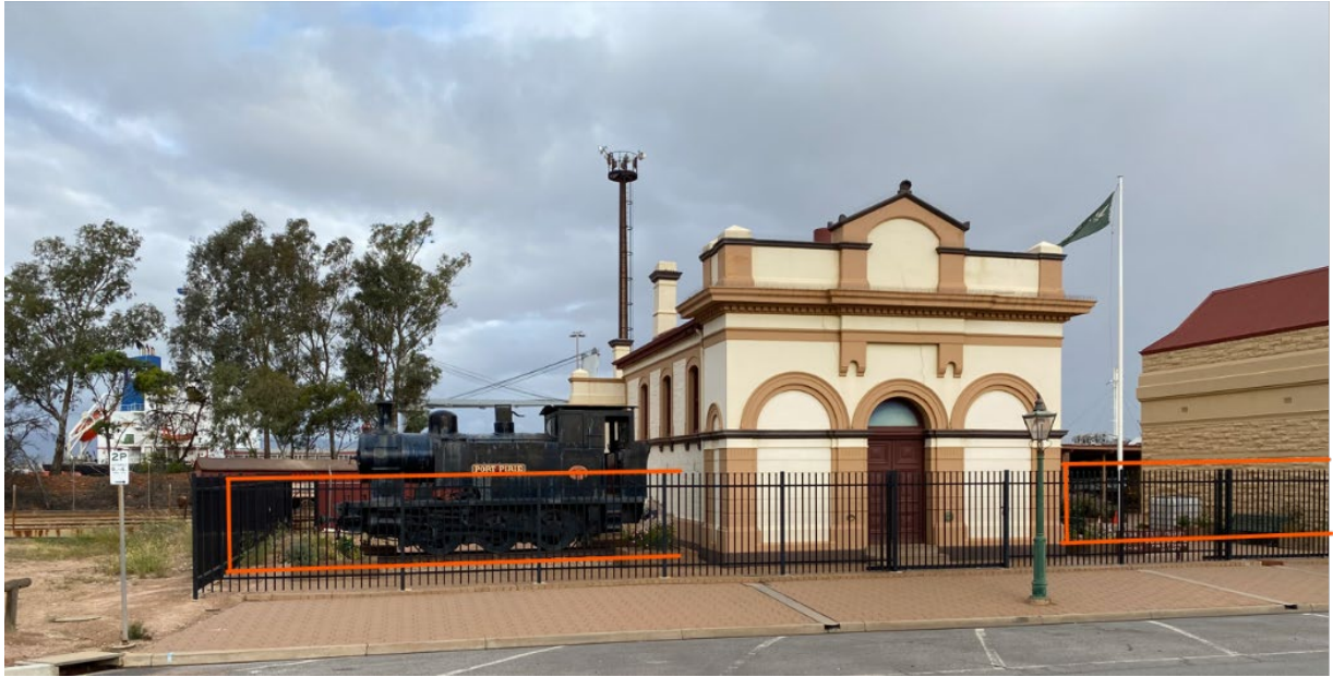
Figure 7: Existing non-original black tubular fencing that detracts from the Former Customs House. The proposal is for new fencing to be set back behind the west façade (shown orange) will allow the façade to become directly connected to the street and become part of the public realm.
