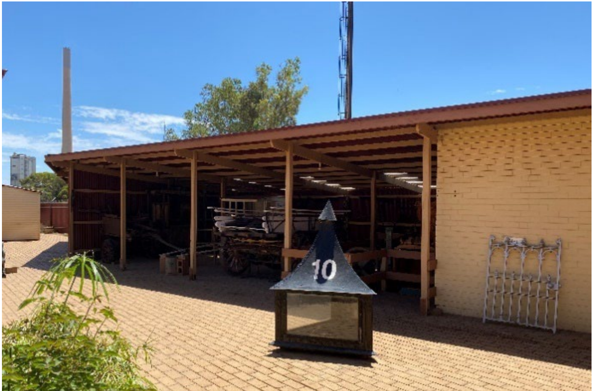
Figure 6: Existing post 1970s non-heritage listed shelter and toilet/storage building proposed for demolition
