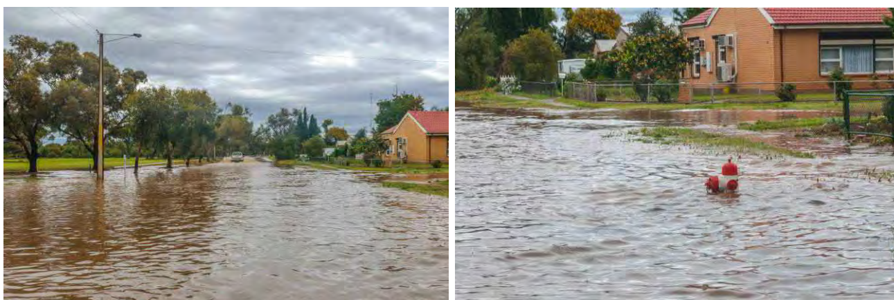
Figure 2.12 Flooding in McLennan Avenue in September 2016 (Whyalla News 30 September 2016)
