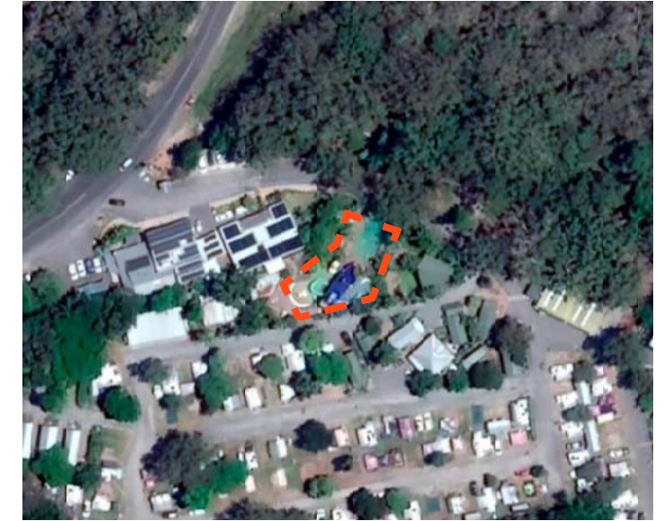
Shipwreck Island Playspace - NRMA South West Rocks Holiday Park, NSW - 30 x 17m / 510m 2 approx
