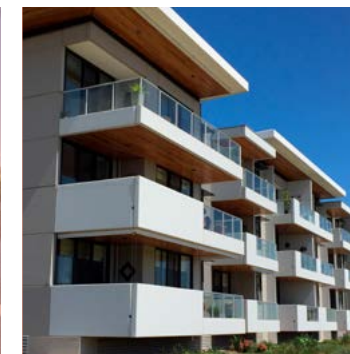
Low-mid level apartment buildings.
