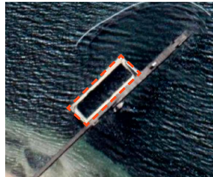
Port Lincoln Swimming Enclosure, SA - 50 x 16m / 800m 2 approx
