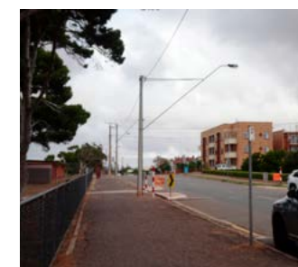
Broadbent Tce looking West.
