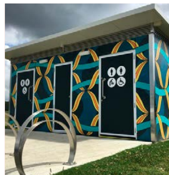
New toilet facilities + amenities.
