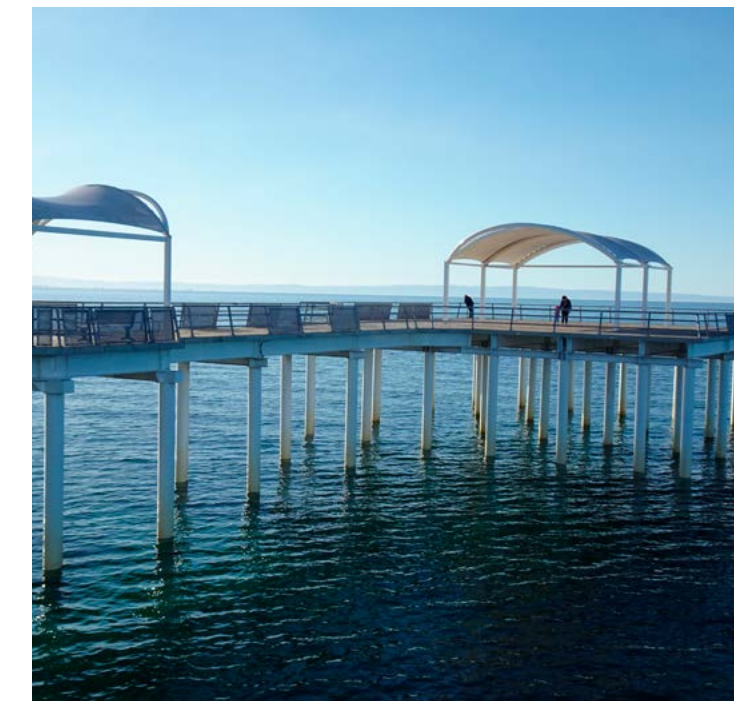
Whyalla's distinctive new jetty with circular walkway is popular with walkers and fishers and was opened in 2020.
