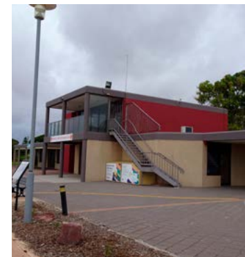
Beach Cafe + SLSC building.
